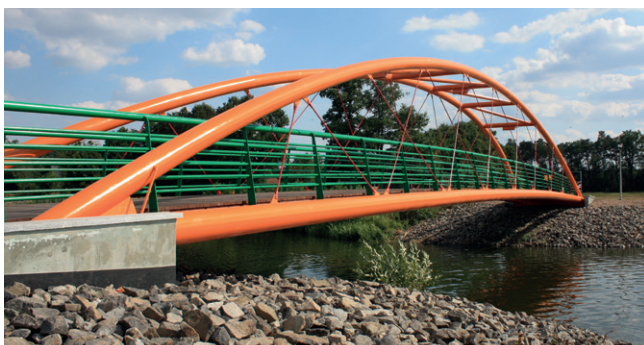
Pedestrian bridge across the laguna at Kluczbork, Poland (Zem Labydy)
