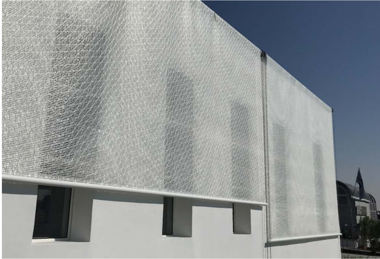
Vertical sun shades on facade
