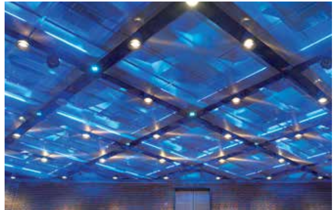
Tonhalle, Dusseldorf, Germany. Architect: HPP Hentrich-Petschnigg & Partner. Mesh: Omega 1540 Bronze (special mesh) (10)
