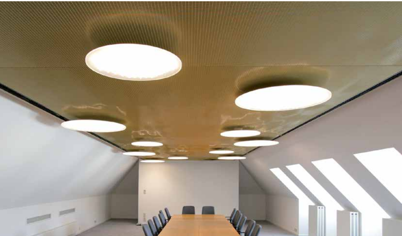
„König von England“ (King of England) Ministry Building, Stuttgart, Germany. Architect: zsp architekten. Mesh: CMP Alu 6010 (7)
