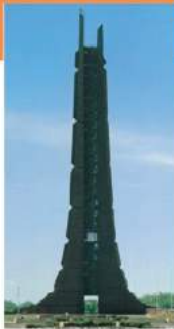
Sep. 1977 (8 years after completion)
