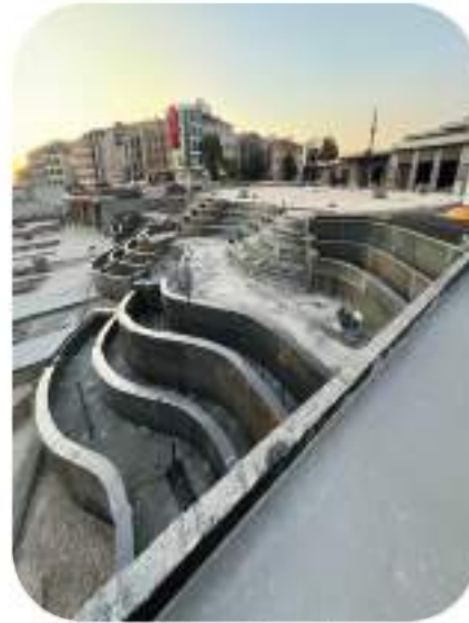
Municipality Building Ankara/TURKEY
