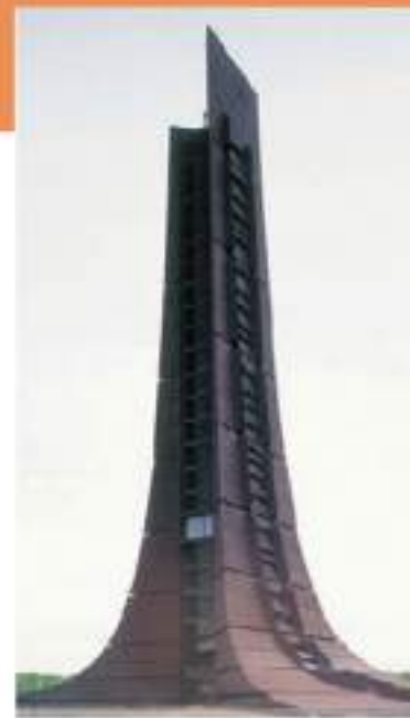
May 1991 (22 years after completion)
