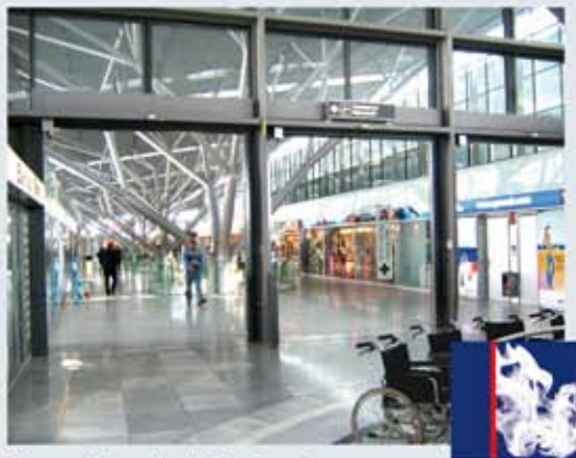
Airport terminal Stuttgart
